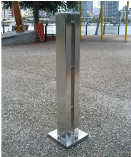
FIGURE 3: Electropolished stainless steel grade 316 in perfect condition after 7 years of exposure in a marine environment.
